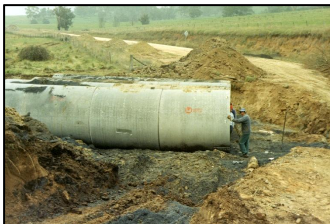
Installing pipes on the Emu Valley Tarana Road. June, 1988
