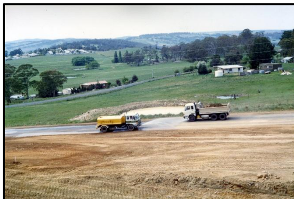
Council road works at the top of Falls Hill, The Reef
